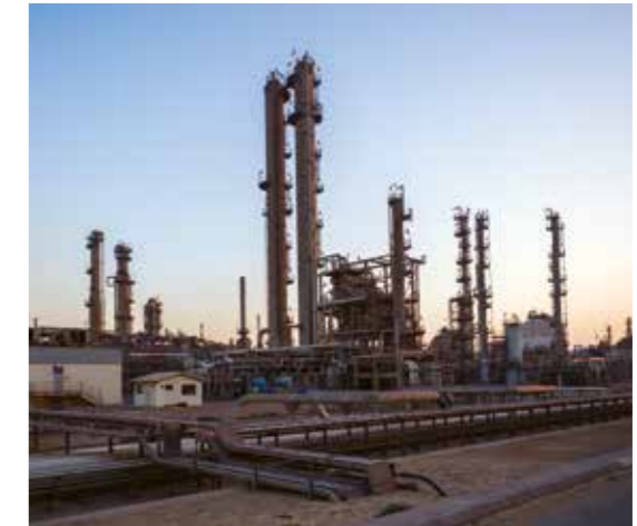
SABIC's Ibn Zahr affiliate cleaned heater coils at its MTBE-2 plant, reducing the site's emissions by 4,300 metric tons of CO 2 each year.
