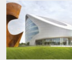
EUROPE HEADQUARTERS Sittard, The Netherlands
