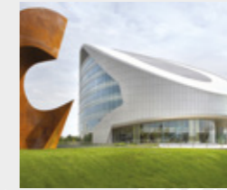
EUROPE HEADQUARTERS Sittard, The Netherlands
