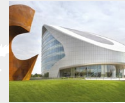
EUROPE HEADQUARTERS Sittard, The Netherlands
