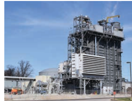
ABOVE Cogeneration unit at Mt. Vernon, Indiana, USA
